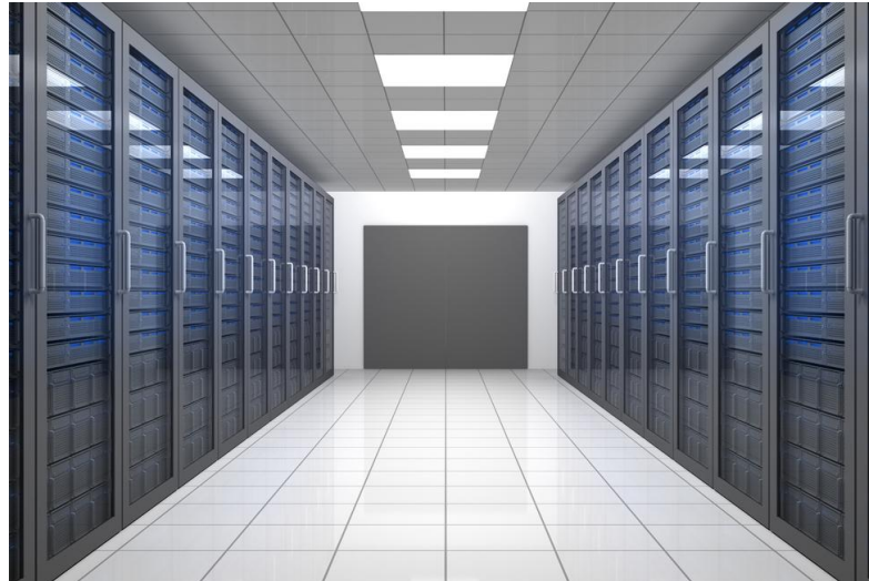
Large datacenter clusters
